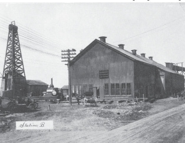
Constructed in 1910 by Western States Electric, Station B operated by primarily burning sawmill waste.
